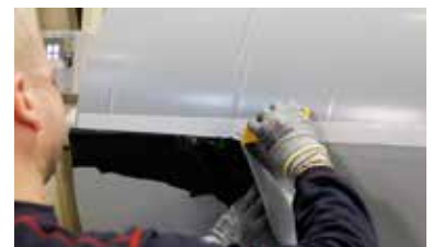
3rd step: Reverse wind substrate back on itself and apply it to the adhesive part. Then remove the overlapping excess substrate.
